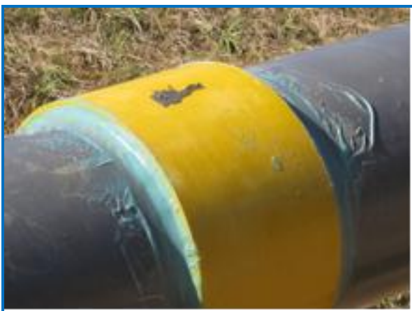
Clock Spring cut to 5 ½" width and installed as casing spacer
