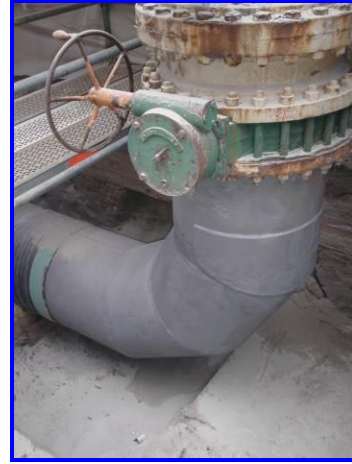
Area to be repaired after sand blasting
