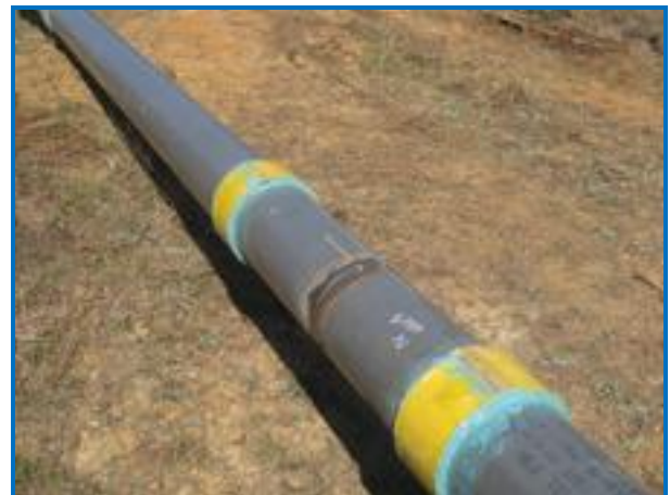
Casing spacers at girth weld joint
