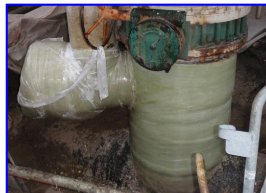
Repair nearing completion
