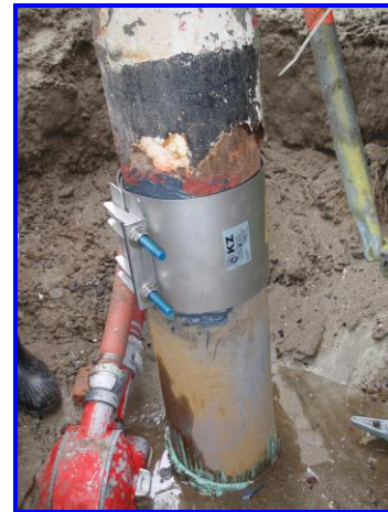
Clamp applied over the leaks and sealed with plastic steel
