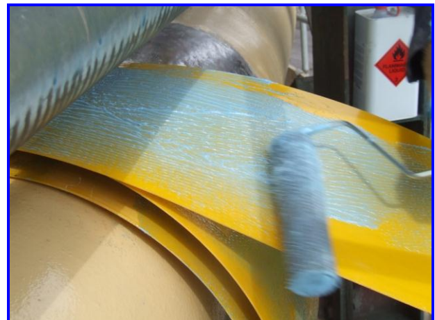
Repair installed using the "hand spool" method
