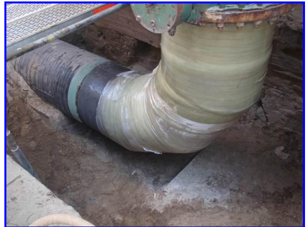
First 4 layers installed and left to cure
