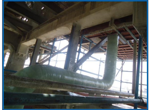
A vertical, horizontal and 2 bends repaired with Clock Spring Contour
