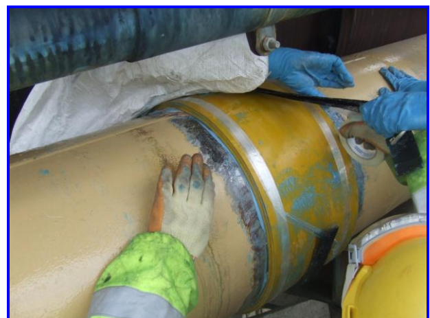
Repair tightened and taped while it cures
