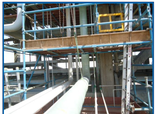
Vertical section of pipe, bend and horizontal section of pipe wrapped with Clock Spring Contour
