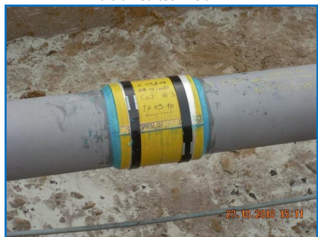
Repair completed and marker bands applied.
