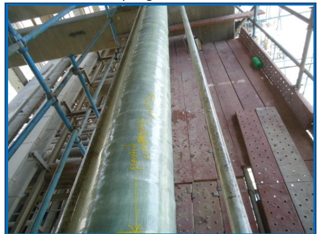
A straight section of pipe wrapped with Clock Spring Contour
