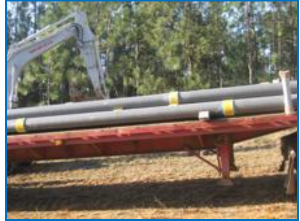
Clock Springs pre-installed on pipe sections
