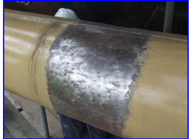
Defect and surrounding pipe cleaned to S.T. 3
