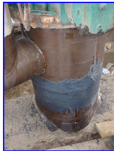
Plastic steel used to seal leaks and taper any sharp gradients
