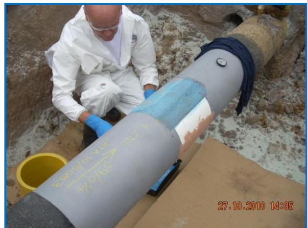
Installation of the Clock Spring Composite Sleeve using a trained technician.
